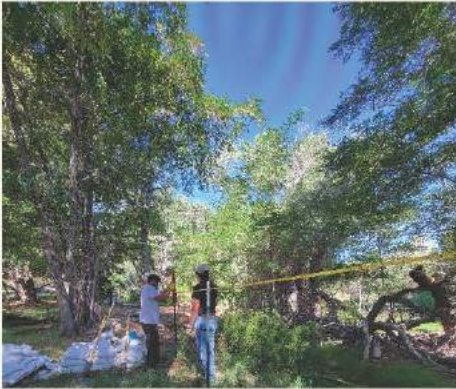
Figure 3: The WQCP with the help of other EMO and BLM staff installed and repaired 80+ feet of cattle exclusionary fencing to mitigate nonpoint source pollution on the Reservation. Jared and Natural Resources Intern, Chaaden, installing T-Posts for the fencing project.
